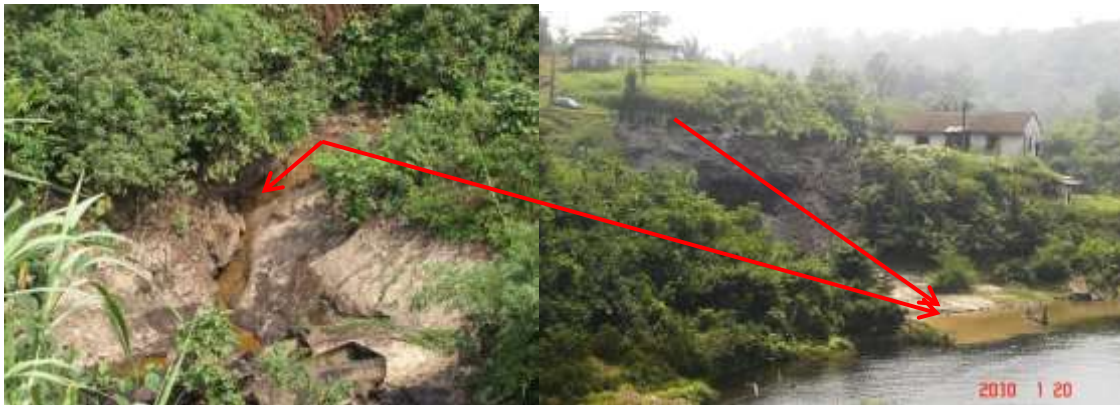
Photos 18 a&b : Pouring of palm oil refinery waste from the PAMOL mill in the Mana River (Ndian basin).
